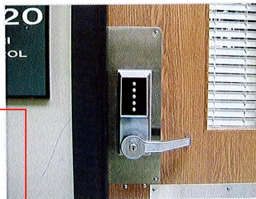
MRI suites should be provided with access controls to keep unscreened or untrained persons away from the hazards.
